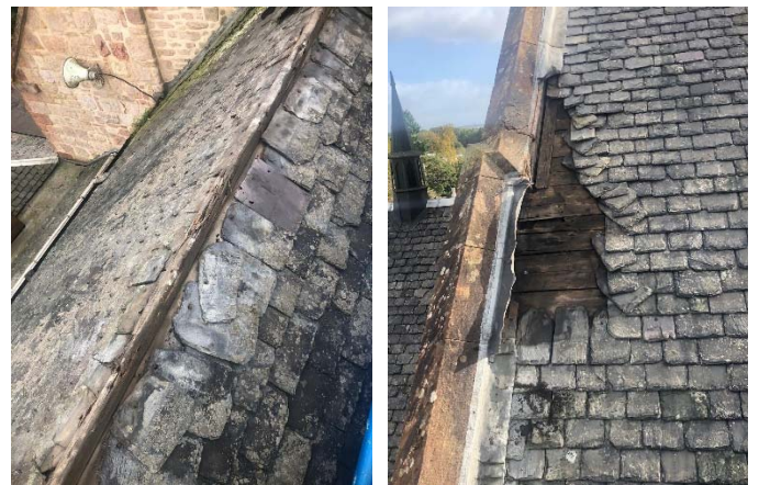
Recent church roof repairs
